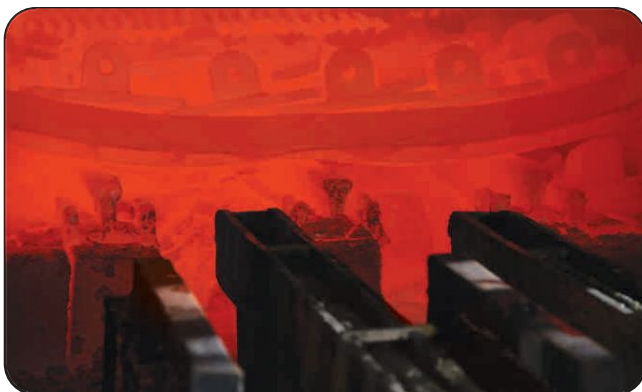
Link Hardening & Tempering Facilities
